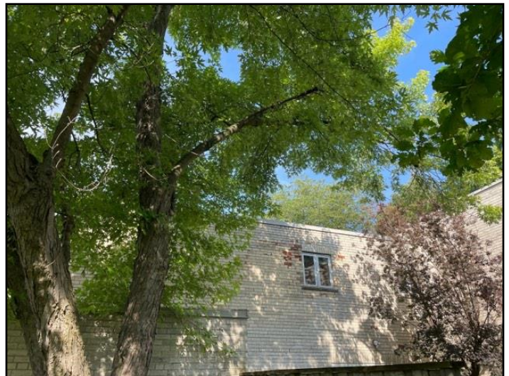
Trees - too close to building...
