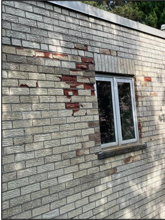
Masonry deterioration
