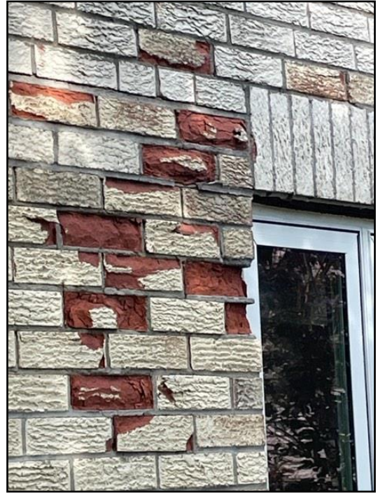
Masonry deterioration
